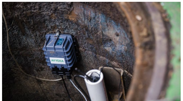
Installation of Wavelet Sewer Overflow Kit in San Francisco, CA
